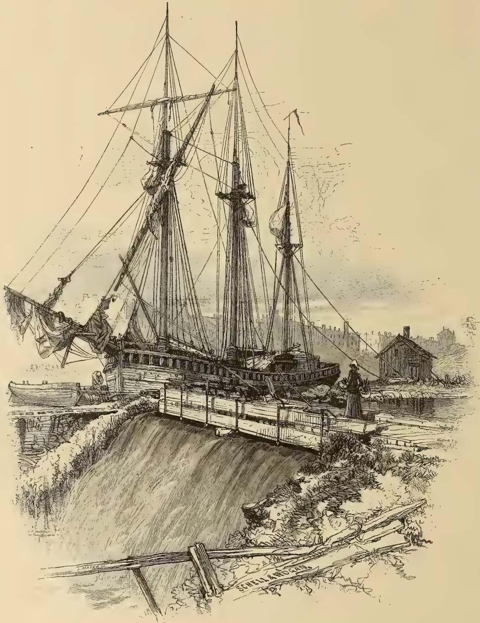
A WASTE WEIR.
